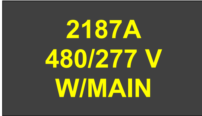
Figure 16. Distribution panel with main power source entry plate/label; 7/8-inch-high yellow letters on 4-inch high by 7-inch-wide black background (figure is approximately 1/2 scale)
