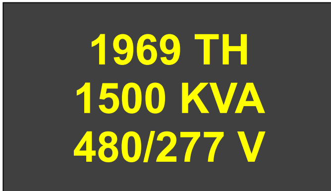
Figure 21. High-voltage transformer label.
