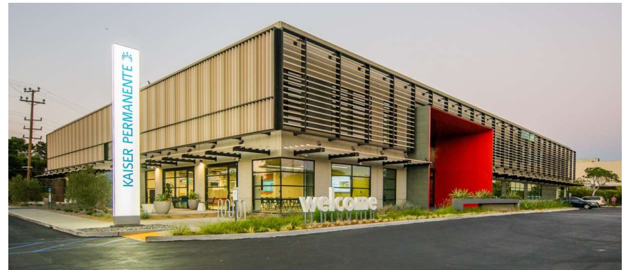
Playa Vista Medical Offices
