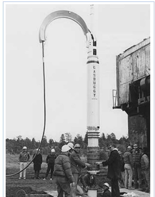
Project Gasbuggy was a stimulation of natural gas production via a nuclear explosion, which took place on Dec. 10, 1967.
